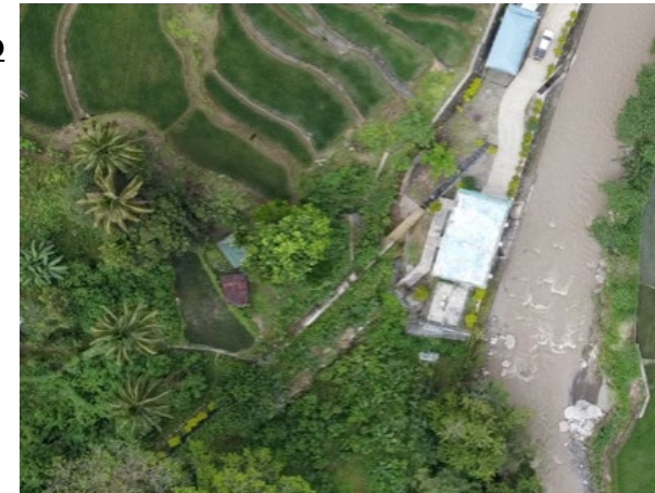
Constructed Likud Mini-Hydro Power Plant
